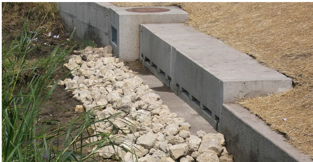
Level spreader outlet structure at Heritage Park in Minneapolis, MN. (photo courtesy - Mississippi Watershed Management Organization mwmo.org )
