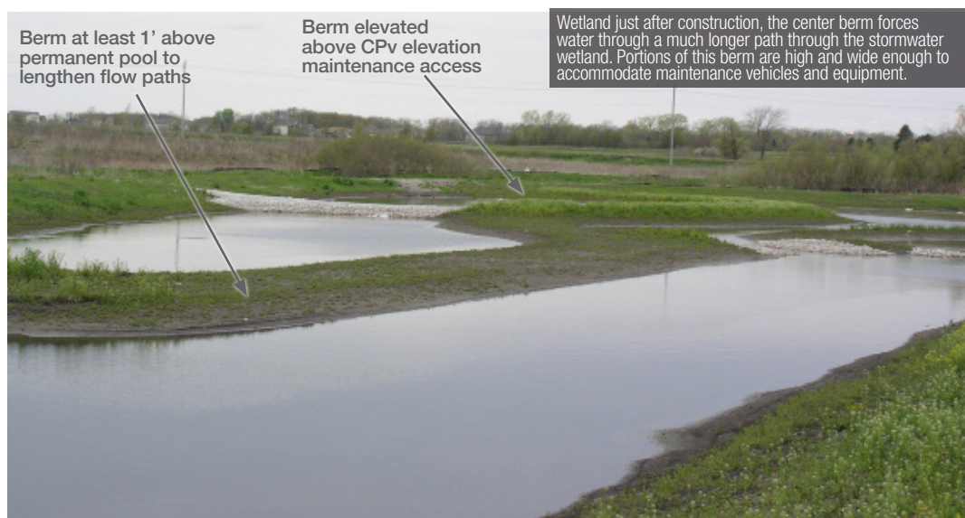
FIGURE 9.08-1-10: TOPOGRAPHIC ZONES WITHIN A STORMWATER WETLAND
