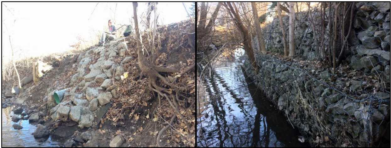
Figure 42. The image on the left shows a poor example of bank stabilization, where debris and cement was slopped into the stream and down the bank. Concrete is not a good way to stabilize it gives no movement for the stream and will speed up the waters movement causing more erosion to occur. The image on the left is between UNI's campus and College Street where apartments are being built, these apartments are right on the streams edge and rip rap was implemented to control bank erosion throughout this area. This kind of stabilization will help to prevent erosion, but not allow the steam to move at all.
